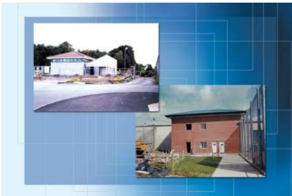
Castlerea Courthouse & New Gatelock under construction at Castlerea Prison
